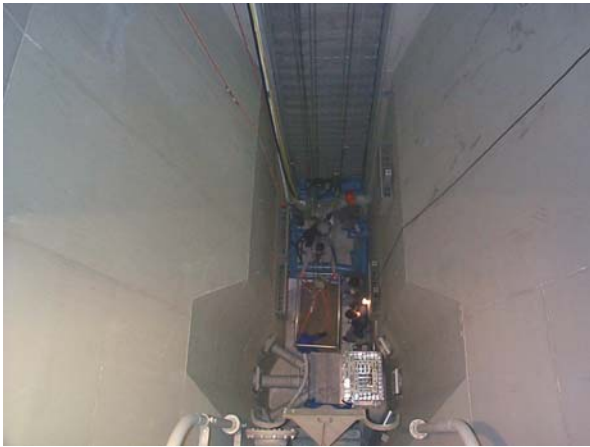
Figure 1 - Looking 30' down into the drained reactor end of the tank. The reactor has been moved to the isolated end beyond the top of the picture.
