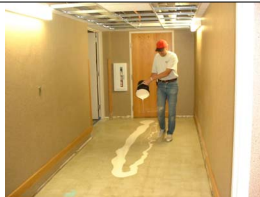
Photo 2 – Pouring the Base Coat
