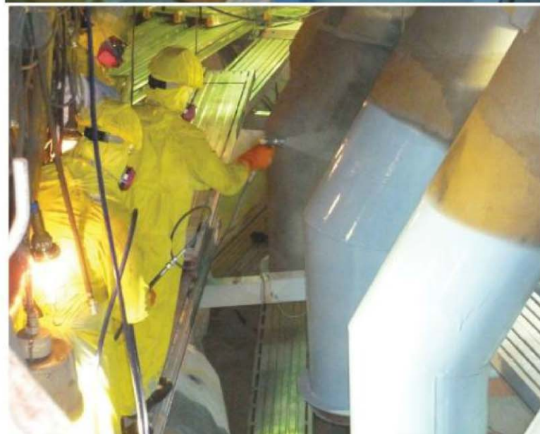
Williams Specialty Services was called in to re-line 32,000 square feet (2,973 m 2 ) of a North American power plant. It had a remote location and angled surfaces: complications this 40-person crew could handle.
