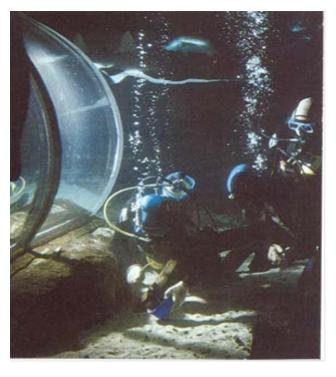
**RESULT:** BIO-DUR 561 has a long track record of successful underwater applications to ship hulls, piers, pipelines and similar structures. In this instance BIO-DUR 561 enabled a neat, professional underwater repair from the "pressure-side" of the leak with no disruption to the normal activities of the facility and with no discomfort to the animals.
