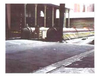
The BIO-FLOR 182 installation was **RESULT:** made well within the time allowed and was ready for unrestricted service about 12 hours after the last application. The surface is seamless, glossy and slip-resistant and has proven a positive barrier to plant chemicals.
