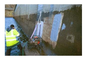
Roller applications of 10 sq.ft. each were carried out immediately after water jetting at ambient temperature of 45°F while the surface was still running wet. To compound the wetness, it was raining heavily during the application and subsequent curing period.
