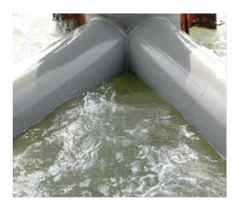
Work started during the end of the hot summer season and continued into the much colder winter. As water temperatures plunged the BIO-DUR 561SW began to increase in viscosity. Thin Film Technology laboratories responded by formulating a lower viscosity "Winter" quality to allow applications well into the cold weather conditions.
