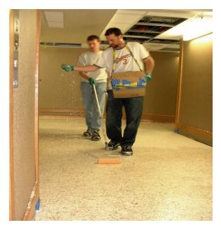
After the "Chip Coat" has cured for about 4 hours a final thin Glaze Coat of BIO-FLOR 182 Clear is applied. The floor is ready for unrestricted service after curing for about 12 hours at 77'F.
