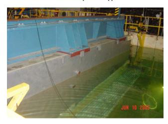
**RESULT:** The coating cured to a "firm", condition within 3 hrs. and was fully hard and tightly adhered after 12 hours. The operation proceeded on schedule and has set the standard for similar future projects.
