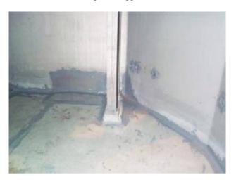
**RESULT:** The BIO-DUR 561 coating was applied by university personnel to selected portions of the aluminum liner including weld seams along the pool floor, around beam flanges, and on several areas of pitting.
