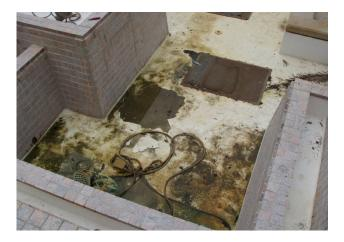
**THE SOLUTION:** TFT created a UV stable version of BIO-GARD 251 in the bright blue color as specified. The thixotropic viscosity of BIO-GARD 251 makes application by brush or roller especially easy. This enabled the Poly-Tuff application technicians to produce a very neat and attractive end result notwithstanding the difficult initial condition of the fountain.
