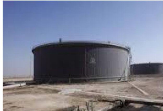
Crude Oil Storage Tank – “COST”
