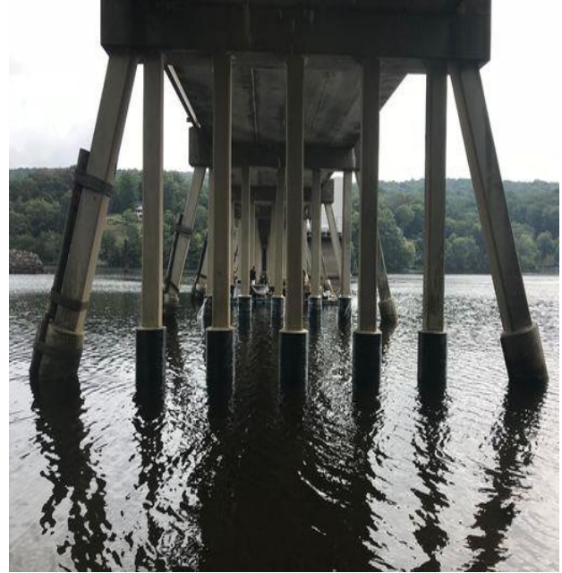
Bridge support repairs – above and below water
