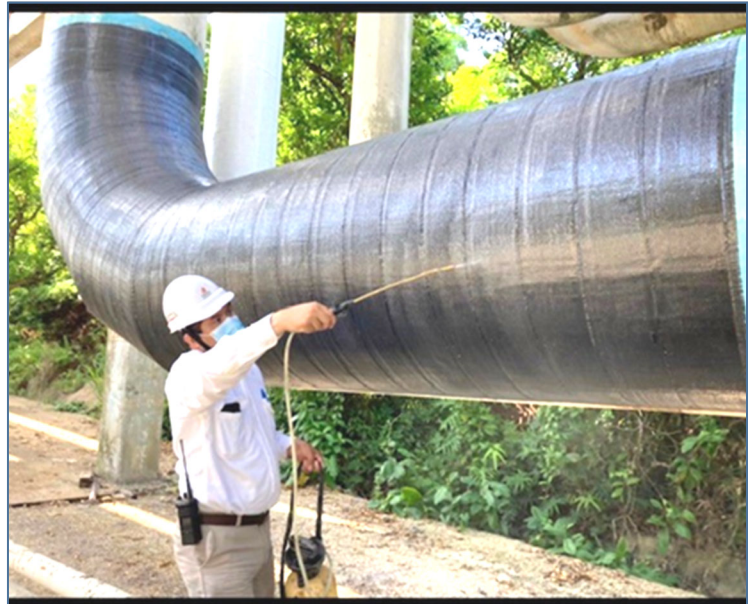
Inspecting carbon fiber repair of pipeline.
