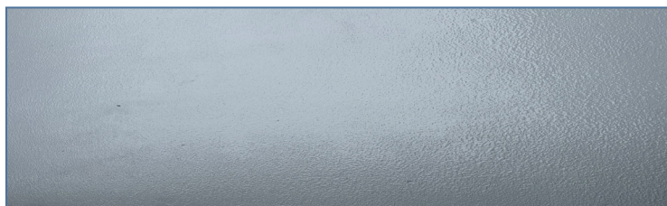
Coated concrete with (2) coats of Bio-Gard 255 and non-skid
